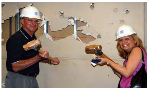
Terry and Paulette breaking ground, looks like a wall?
